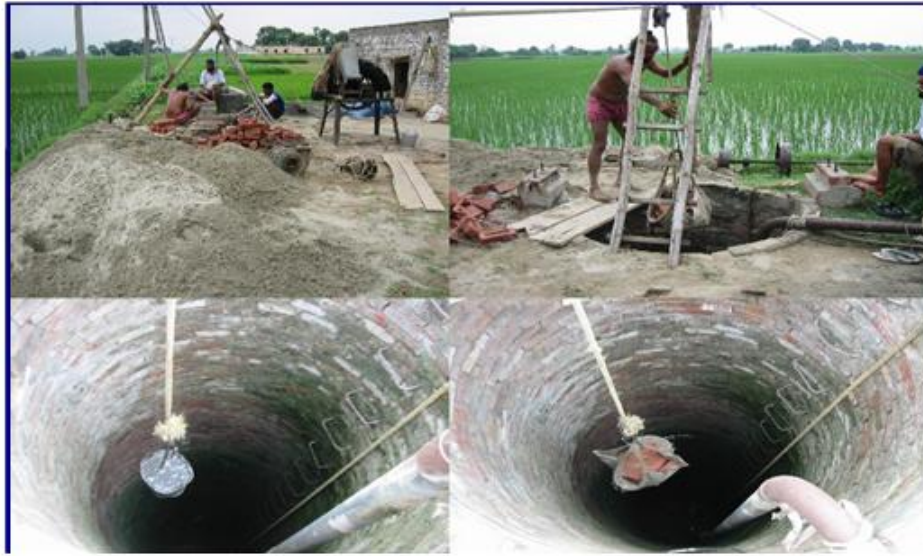
Fig. 1. Deepening of the bores of the tubewells because of declined underground water table
