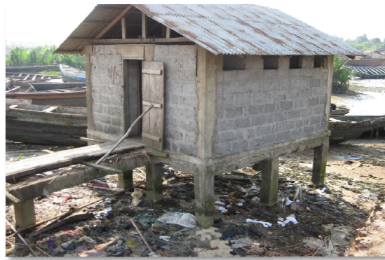
Plate 2. A typical latrine in Ibaka where deposited excreta was carried by receding tide
