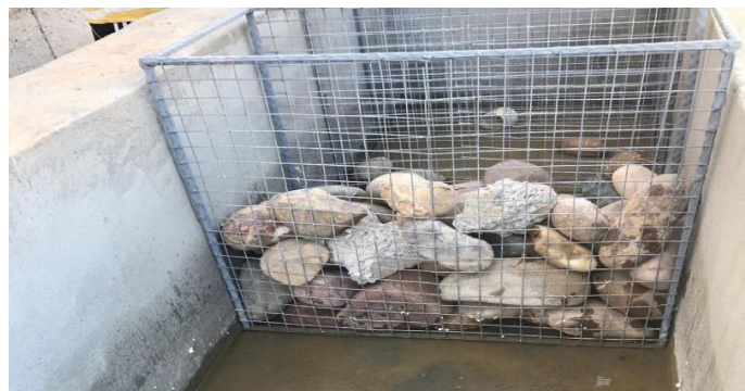
Fig. 5. Interceptor dike to control the erosion
