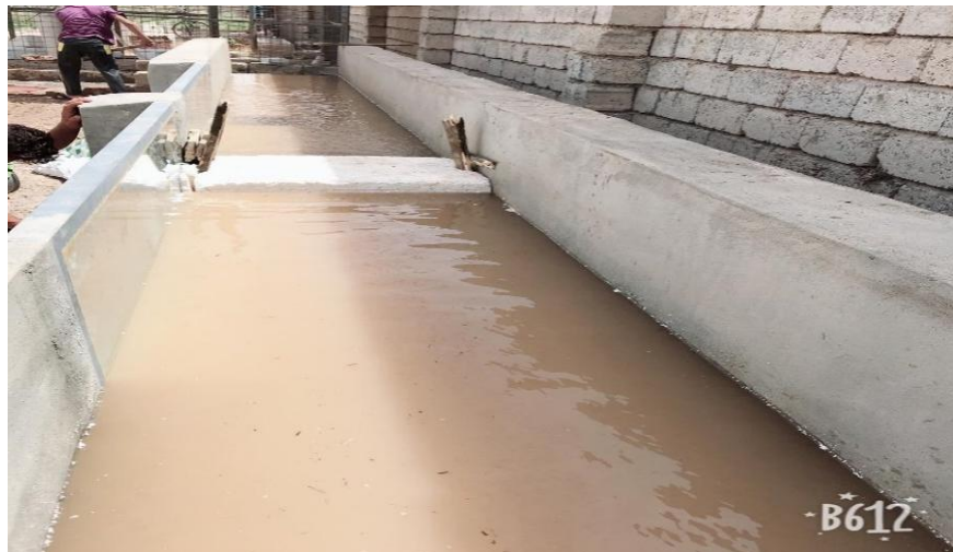
Fig. 9. The Floating Bridge construction
