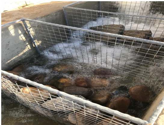
Fig. 3. Cooling pools and flow regulation
