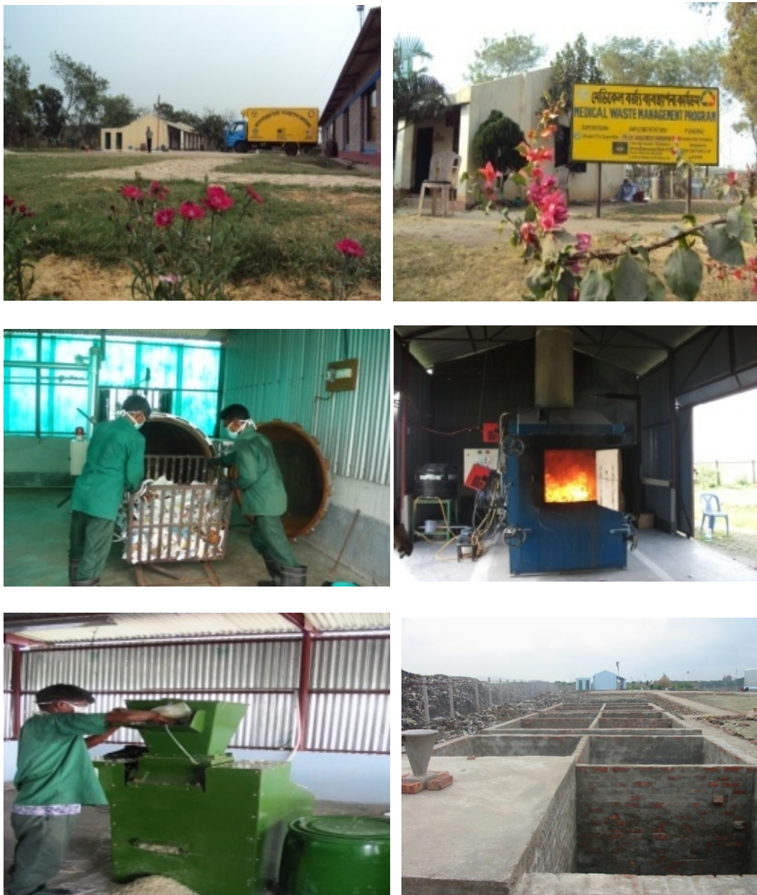
Fig. 4. Matuail treatment centre facilities
